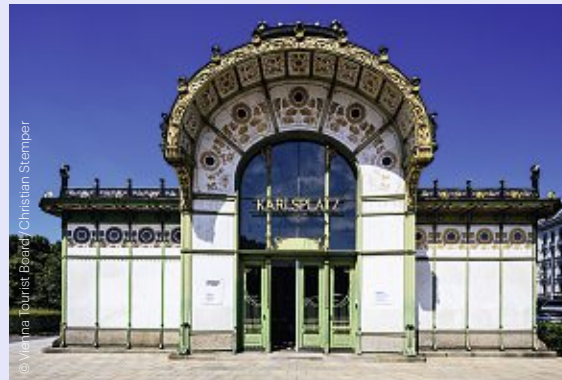
OTTO WAGNER PAVILION ON KARLSPLATZ THE STADTBahn RAILWAY WAS AMONG WAGNER'S PRINCIPAL WORKS
